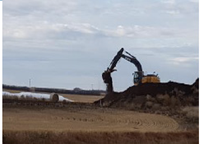
Excavator pulling topsoil back on ROW – SF 79 - Oct 30, 2018
