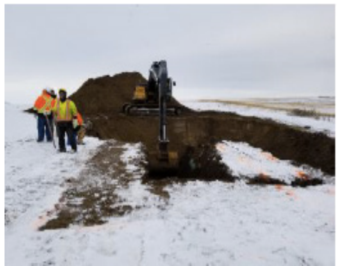
Excavator digging to expose pipe – SF 44 – Nov 3, 2018
