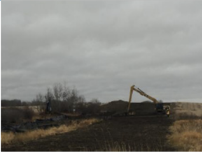
Excavators replacing topsoil – SF 51 – Nov 1, 2018
