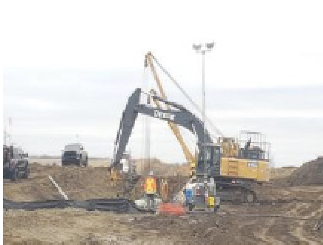
Crew working on tie-in - SF 34 – Nov 1, 2018
