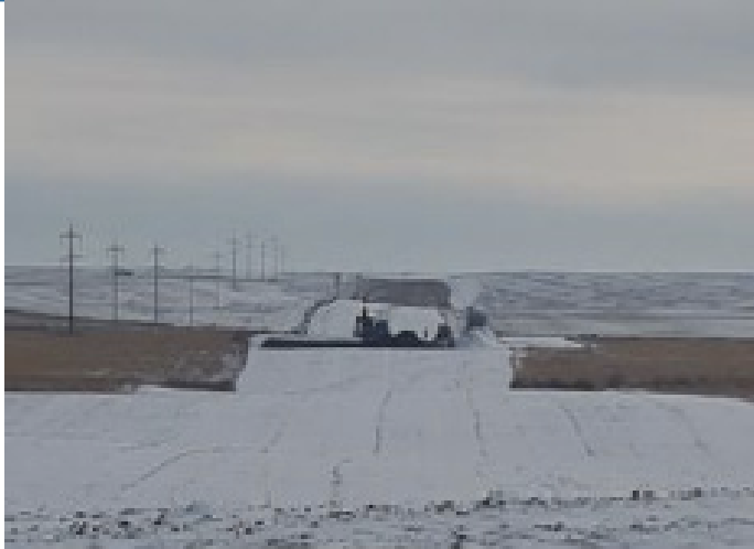
Equipment working on ovality dig - SF 40 – Nov 3, 2018
