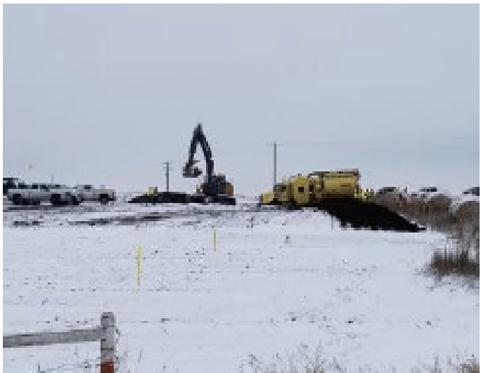
Hydrovac prepping to day light pipe - SF 46 – Nov 3, 2018
