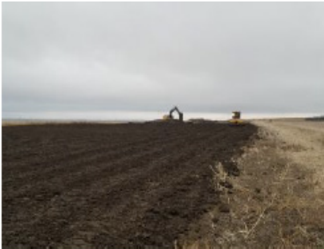
Topsoil placement– SF 66 – Nov 1, 2018
