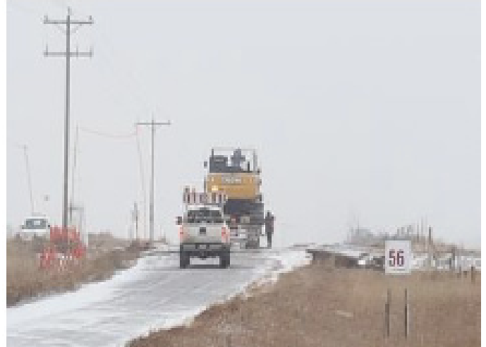
Lowboy transporting excavator – SF 56 – Nov 2, 2018
