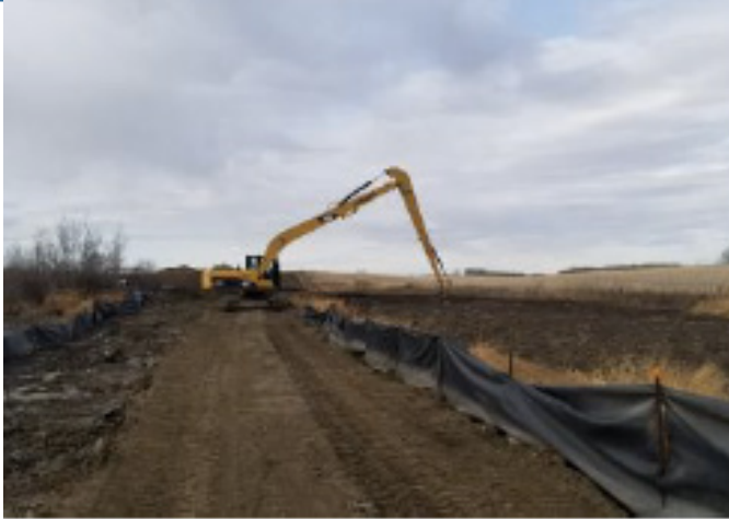
Excavator fixing roach on wetland – SF 52 – Oct 31, 2018
