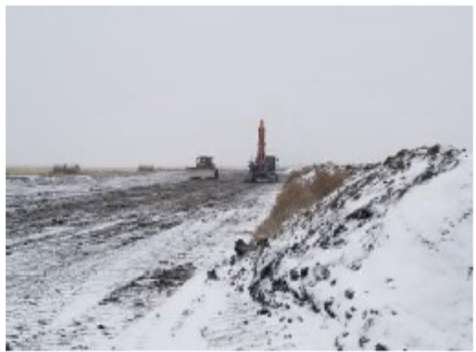
Equipment track packing subsoil – SF 44 – Nov 2, 2018
