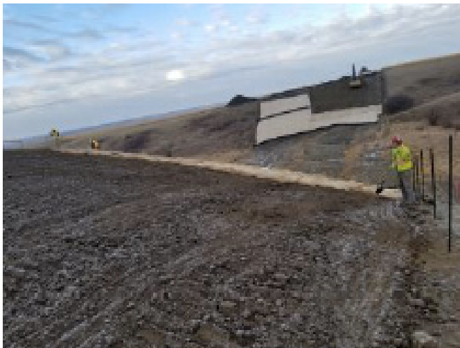
Crews placing mats for erosion protection – SF 70 – Oct 30, 2018
