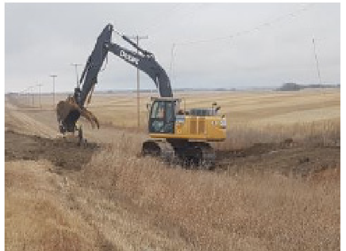
Excavator working on ramp removal – SF 78 - Nov 1, 2018
