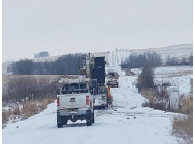
Lowboy transporting excavator off of ROW– SF 52 – Nov 3, 2018
