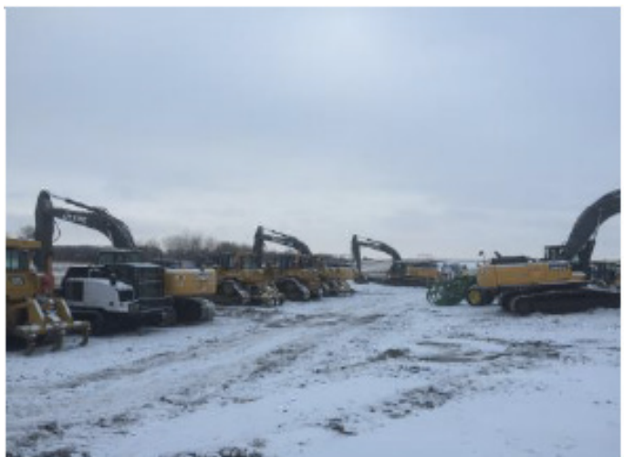
Equipment(18) to haul - SF 52 – Nov 3, 2018
