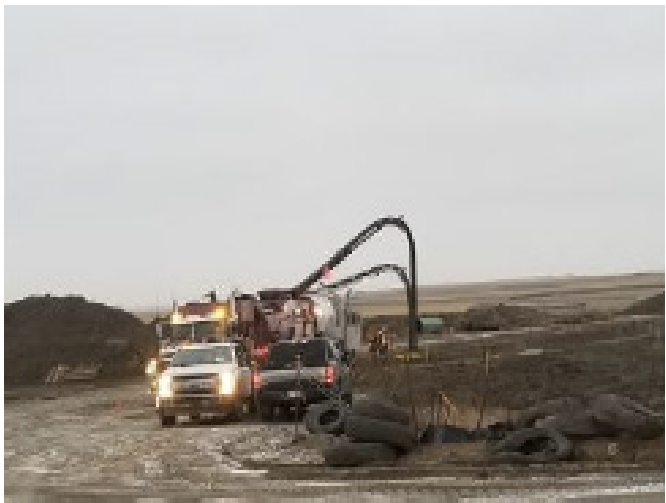
Hydrovacing test sites - SF 72 – Nov 2, 2018
