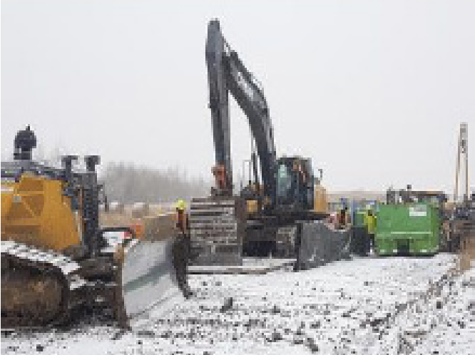
Utility crew cleaning excavator - SF 52 – Nov 2, 2018
