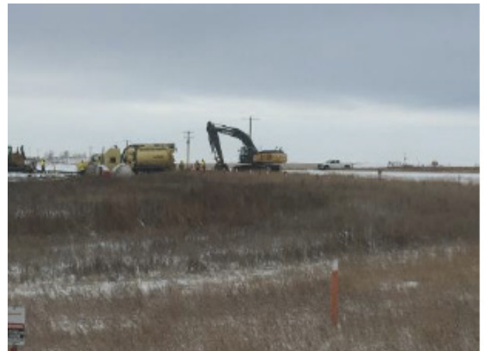
Hydro vac stuck on ROW – SF 45 – Nov 3, 2018
