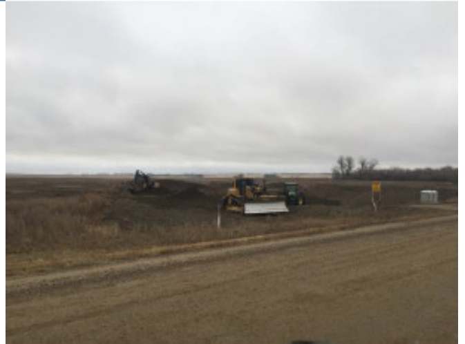
Dozer and excavator on topsoil – SF 77 – Nov 1, 2018
