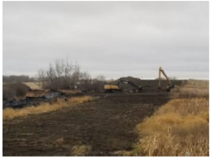
Excavators removing ramp material– SF 52 – Nov 1, 2018
