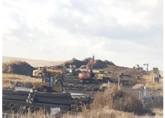
Ramp removal at wetland– SF 44 - Oct 29, 2018
