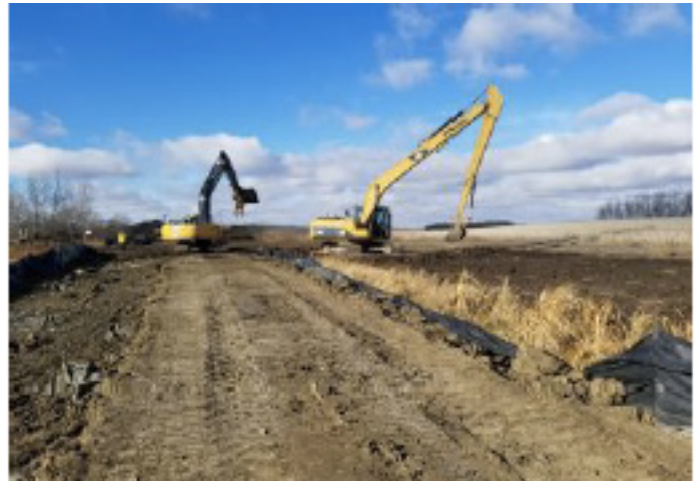
Excavator roach shaping – SF 52 - Oct 29, 2018
