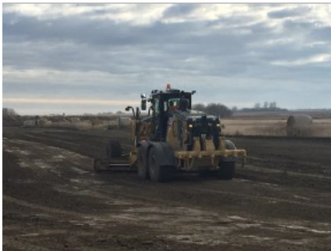
Grader working on transition – SF 77 – Oct 30, 2018
